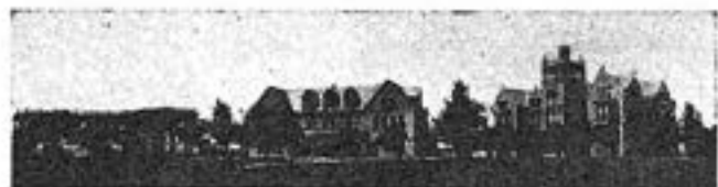
VIEW OF SOUTHWESTERN'S CAMPUS
